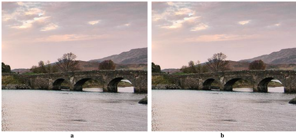
Fig. 3: Before (a) and After (b) the covering process
